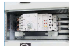
NZM2 circuit breaker with removable neutral link.
