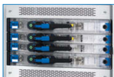
Fused switch-disconnector, form 3b compartment.
